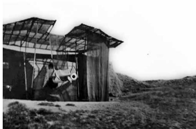
One of the 6" guns at Fan Bay Battery
